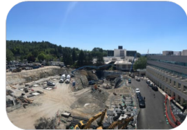
Spring 2019 Building Construction Underway
